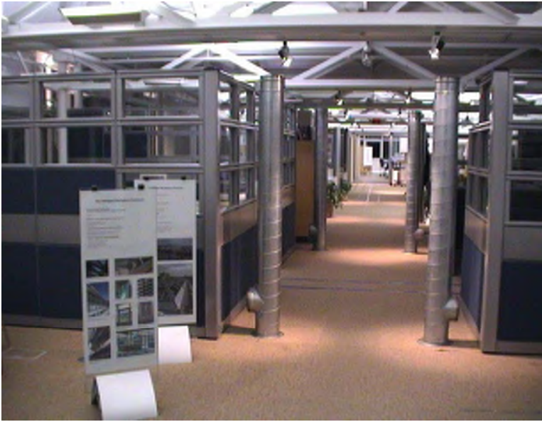
Figure 4.34: The density of return air diffusers and their location directly overhead is key to indoor environmental quality and energy efficiency. In the Intelligent Workplace, return air columns allow the floor to be the sole HVAC distribution layer.
