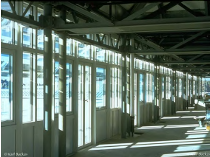
Figure 7.1: The Intelligent Workplace façade integrates water flow mullions for perimeter conditioning.
